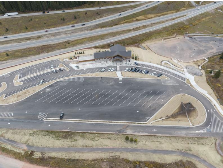
Expanded truck parking at Vail Pass Rest Area
